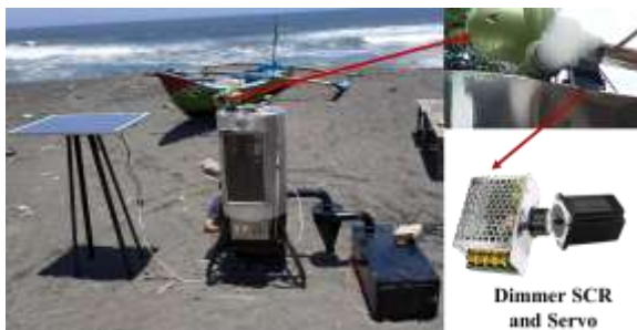
Fig. 9. Blower RPM control system installation.
